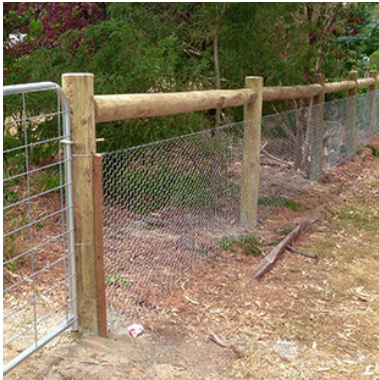
Post and rail fence with wire infill
