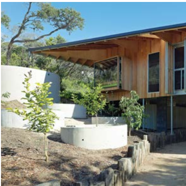
Landform retaining - concrete pipes
